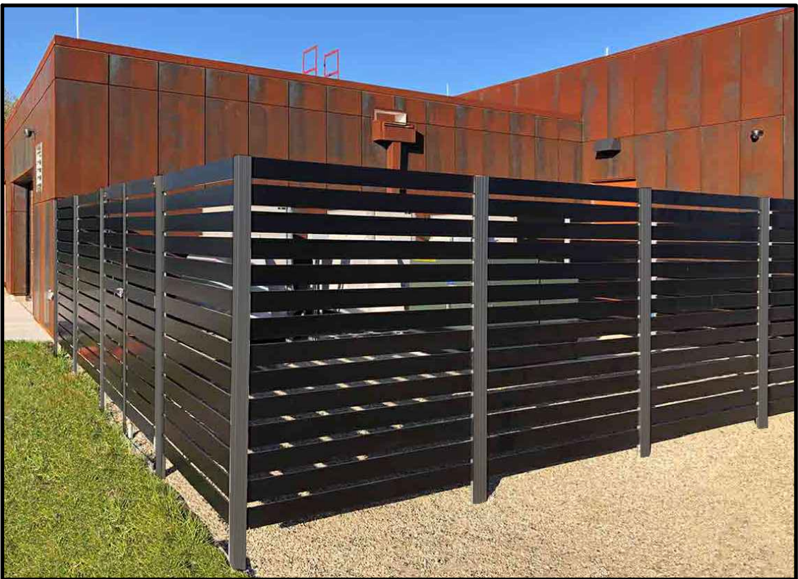
ALUMINUM MECHANICAL SLAT SCREEN FENCE REFERENCE
