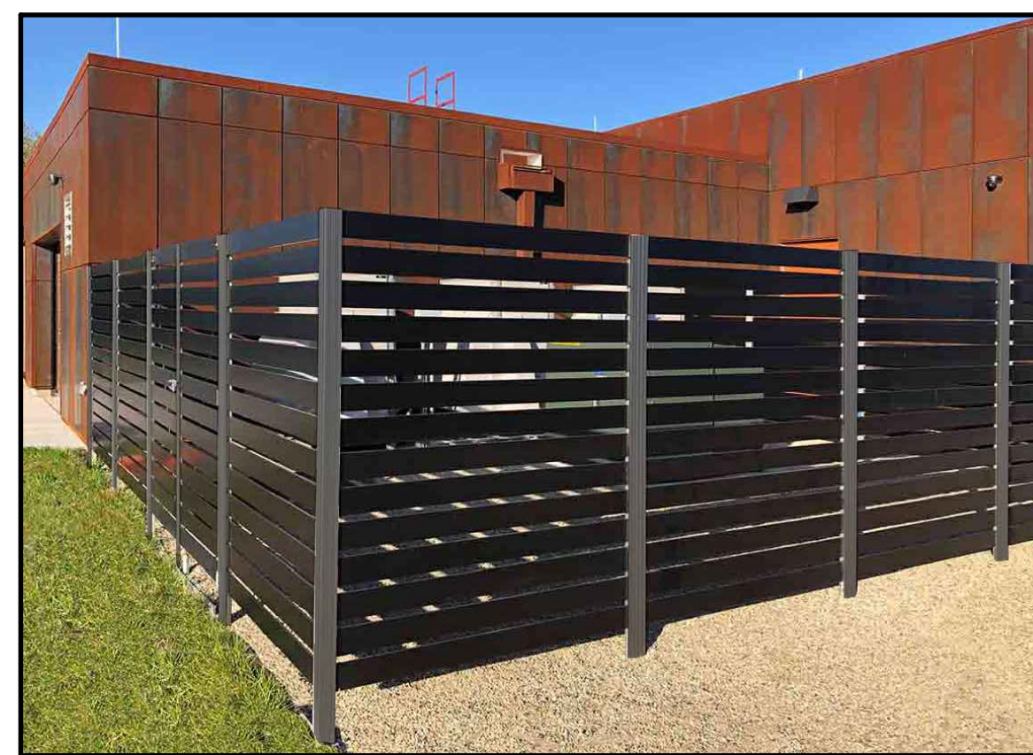
ALUMINUM MECHANICAL SLAT SCREEN FENCE REFERENCE
