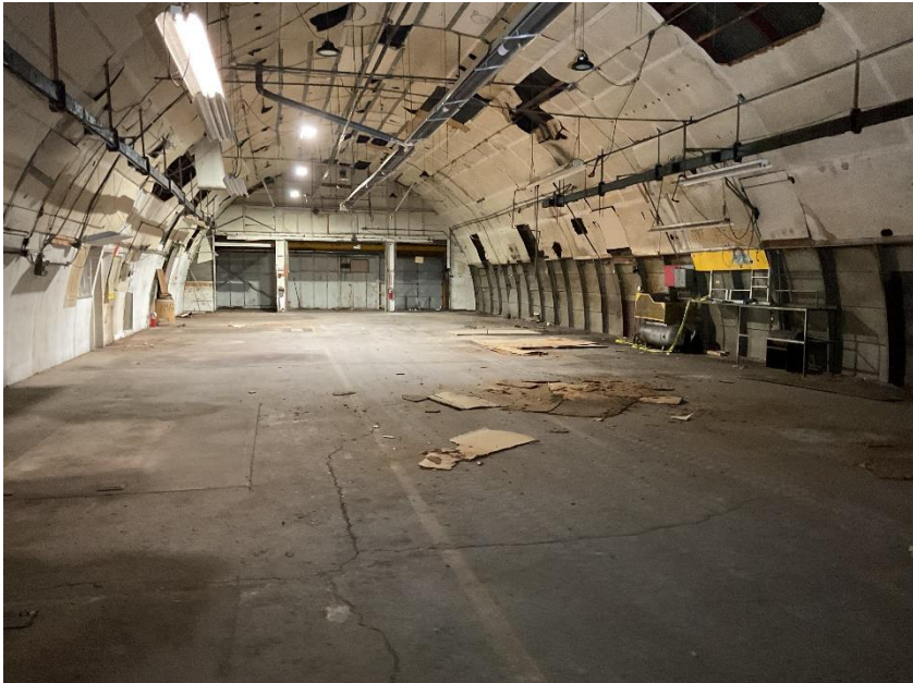
Shop area in the Quonset building in the central portion
