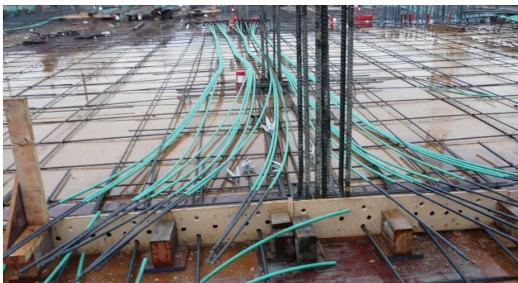
Post-tension cables
