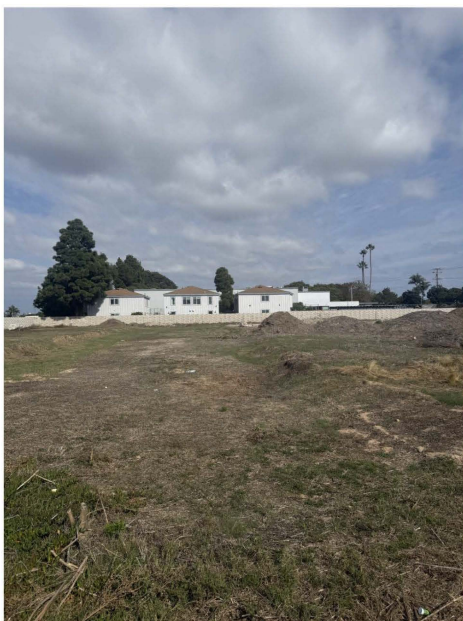
Photo 1: View of Project site facing northeast.
