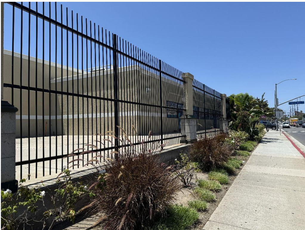
Photo 4 – Former garden center to be removed from Wilson Street
