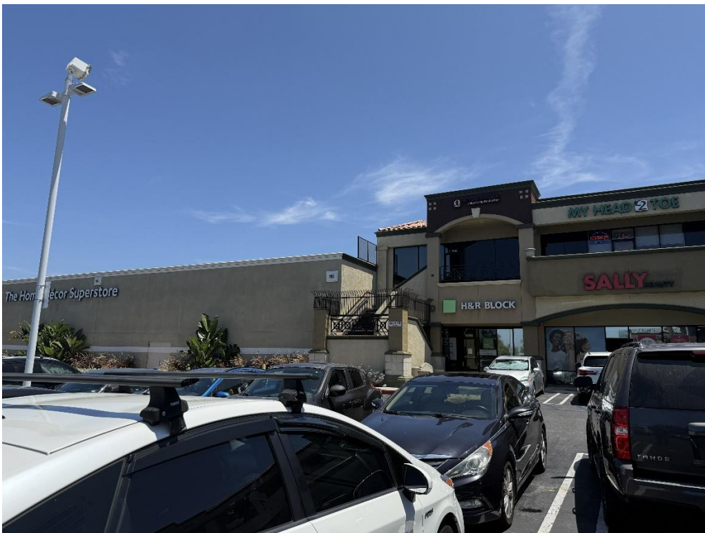
Photo 2 – Height comparison of current structure from parking lot
