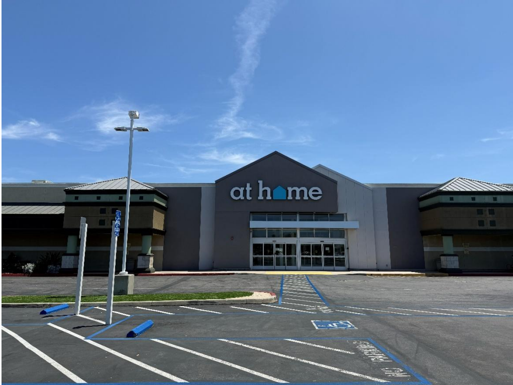
Photo 1 – Existing storefront view from parking lot
