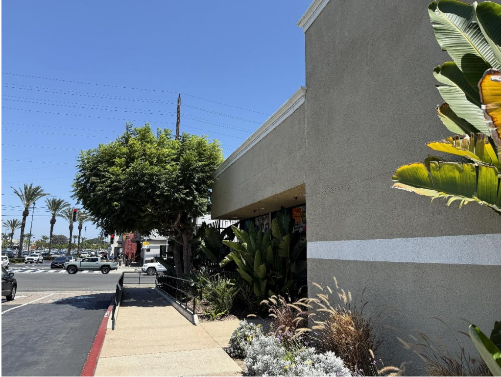
Photo 3 – ADA pathway to Wilson Street from storefront
