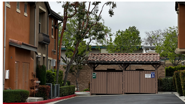
Trash enclosure designed in the same style as primary building.
