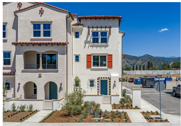
Ground floor residential units with transitional entry spaces.
