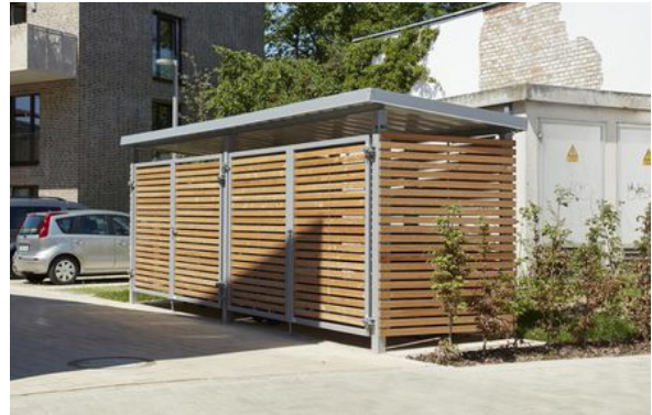
Shared trash and recycling enclosure.
