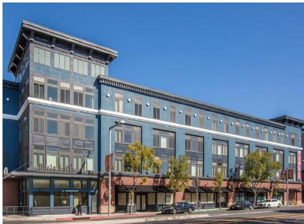
Use of pilasters/engaged columns and change in roof height.
