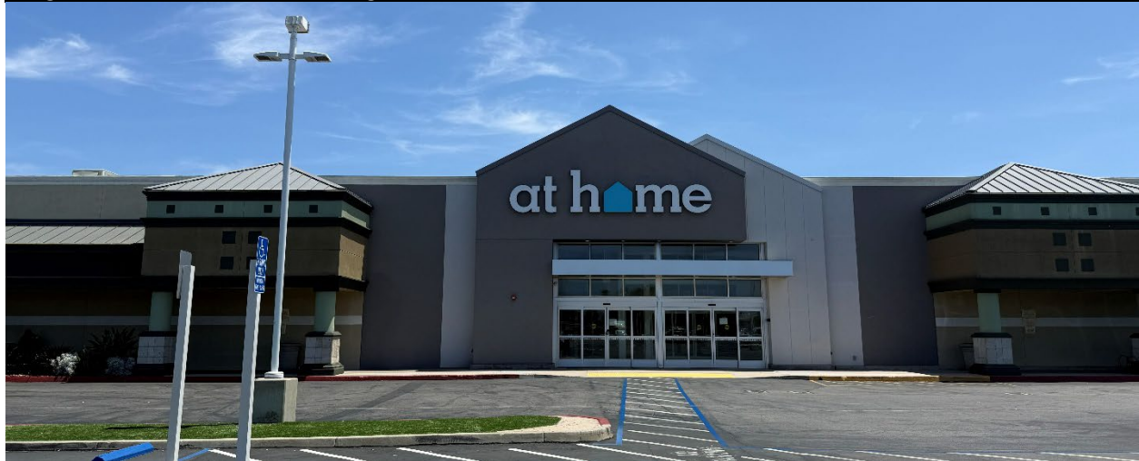
Figure 2 Existing Site Photo - Unit K
